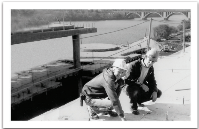
Local 5 members Jimmy Grainer and Bobby Singleton on the site of an early 1980s construction project at The Washington Harbour.
