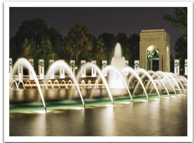
Situated on the National Mall between the Lincoln Memorial and the Washington Monument, the World War II Memorial opened to the public in April 2004. The fountains, a centerpiece of the memorial, were installed by Local 5 members.
